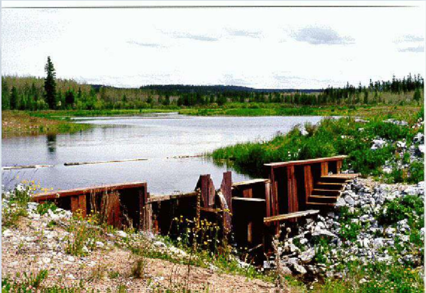
Constructed Wetland Prince George, BC Control Structure
