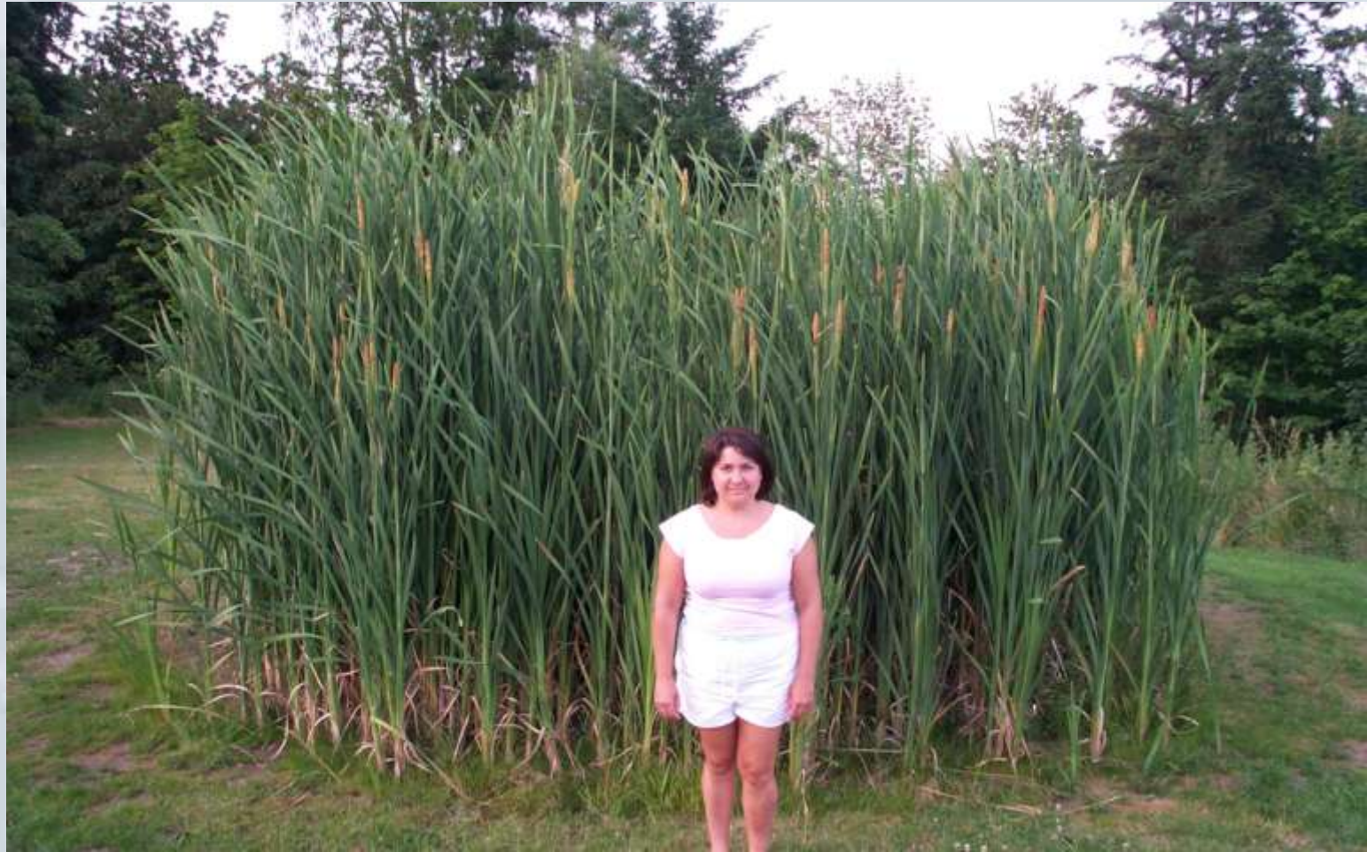
A Proud Homeowner VTF installed on Cherry Point Road, Cobble Hill, BC
