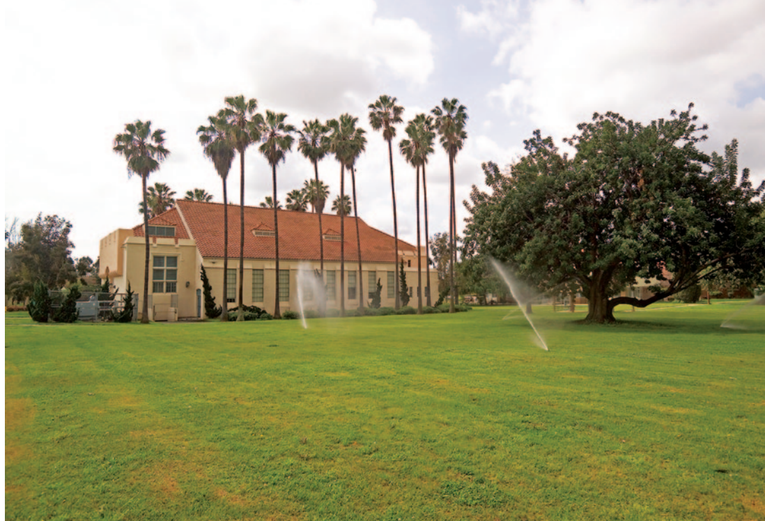
Metropolitan State Hospital uses recycled water for their irrigation. Photo courtesy of Central Basin.
