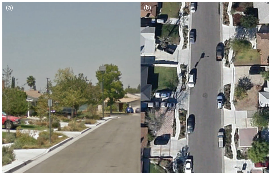
FIGURE 3 | Google earth images showing a network of bioretention units at Elmer Avenue in Los Angeles. This is referred to as a green street. Shape and proximity to other bioretention units or vegetated areas may affect development of plant and animal species that promote desired functions.
